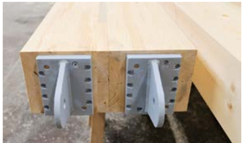
Steel bracing parts, primed and provided with R30 fireproof coating, RAL 7001 top coat
